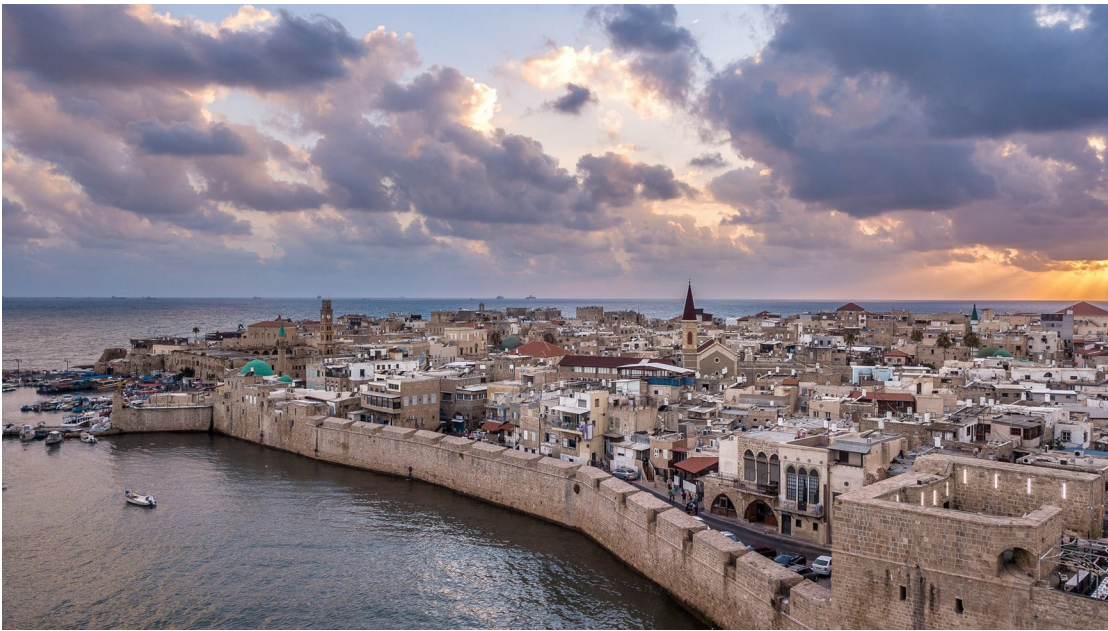
Image description: A panoramic view of Old Akko, its walls, harbor, religious buildings, and dense historic neighborhoods.
